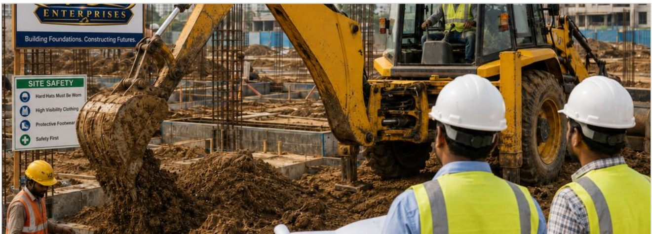
Safety-first practice on every VJ Enterprises site
